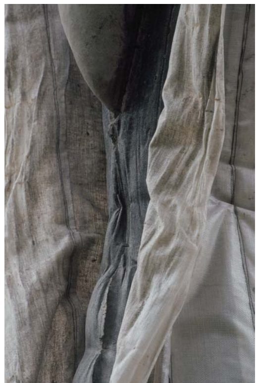
10. Fabric-formed column being unwrapped. Bar Harbor, Maine. 1990
