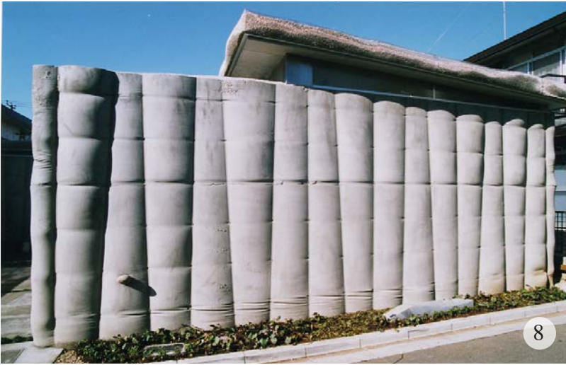
Fig. 8 shows the exterior concrete walls of Unno's "Stone renaissance" house, built in Funabashi City, Chiba for Susae Nakashima (2005). These walls are constructed using steel pipes restrained by standard form-ties running through holes drilled in the pipes. The (slightly diagonal) vertical impressions left by these pipes are freely composed as part of the wall's design.
