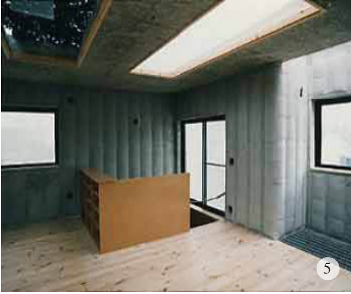
Fig. 5 is an image of the first building 2 constructed with cast-in-place fabric-formed walls. The two skylights shown are experimental passive (evaporative) cooling devices: the one on the right containing water, and the one on the left containing water-soaked charcoal (to increase the rate of evaporation).
