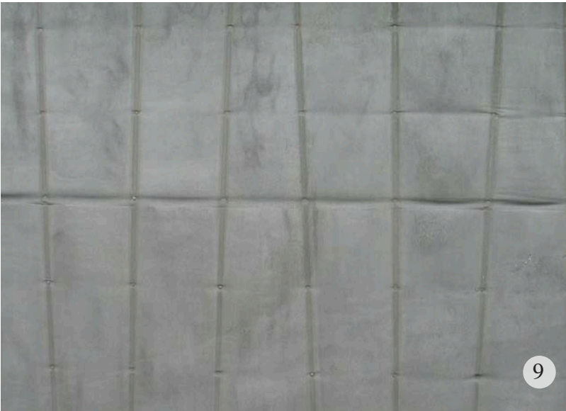
Fig. 9 shows a close-up of the Nakashima "Stone Renaissance" house walls. The horizontal depression running along the length of the wall, just above mid-height, is given by the horizontal overlap of upper and lower sheets of netting (this netting comes in approximately. 2 metre-wide roles -- geotextile fabrics come in roles up to 17.5 ft. (5.3m) wide ). The sheets are not fastened to each other along this joint, but are simply allowed to overlap as the pressure of the wet concrete presses one sheet firmly against the other. The form-ties also leave their own slight horizontal 'echoes' in the surface of the pressurized membrane.
